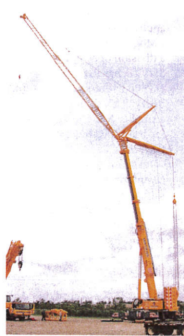
■ Certified Crane and Rigging's LTM 1350-6.1 during commissioning/training.
